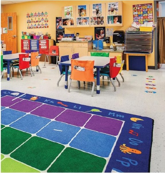
For North Star Early Childhood Educational Center, RMT Construction & Development Group, LLC completely renovated a 39,000-square-foot former church building, transforming the space into new classrooms, a gymnasium, staff areas and a state-of-the-art kitchen and cafeteria.
